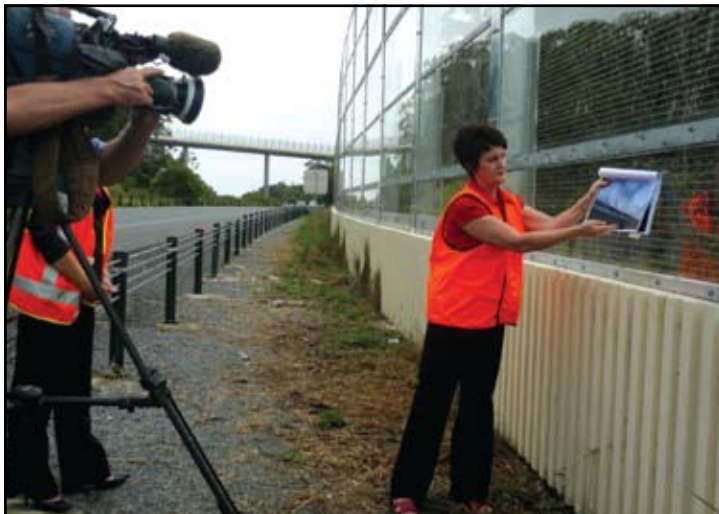
New polycarbonate panels on the Tugun bypass
